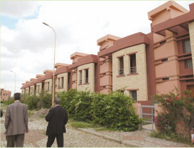
Villa type development at Tamnsourt
