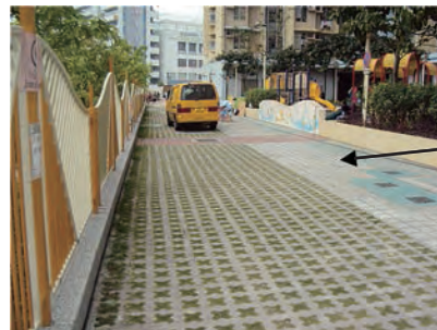
A flat pedestrian route along a 'grasscrete' estate road
