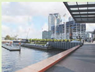
Redevelopment (far end) of the Docklands Area in progress
