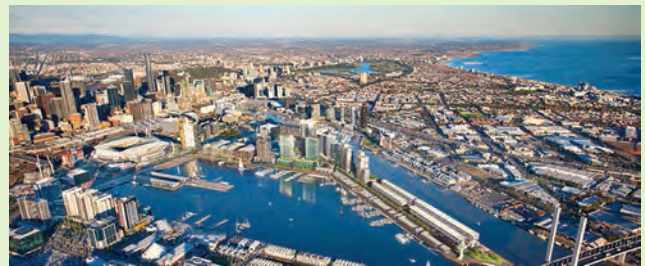
An aerial view of the Melbourne Victory Harbour and Docklands (photo courtesy from Land Lease, Australia)
