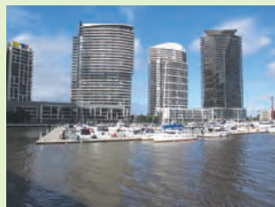
New Residential and Commercial developments along Melbourne Dockland
