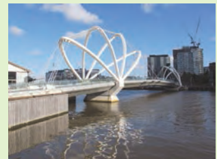
Bridge connection between the North and South Bank
