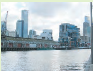
Melbourne Docklands Area – Existing dilapidated wharf structure along the Docklands yet to be redeveloped
