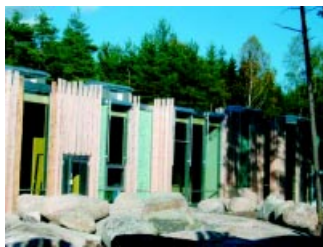
Local and environmental friendly materials employed for the external facade
