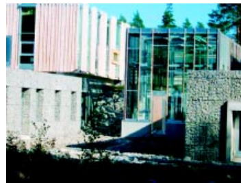
Skylight for natural lighting
