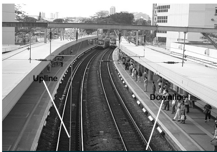
Fig. 1 Kowloon Tong Station monitoring area
