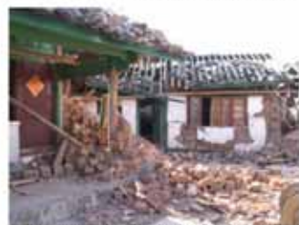
Houses collapsed after the earthquake
